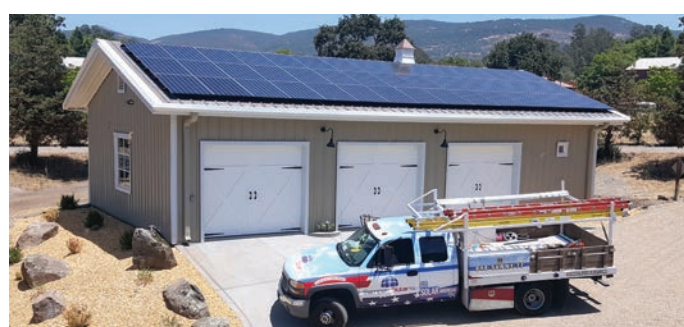
Semper Solaris team installed SunPower® panels, which will produce 70% more energy.
