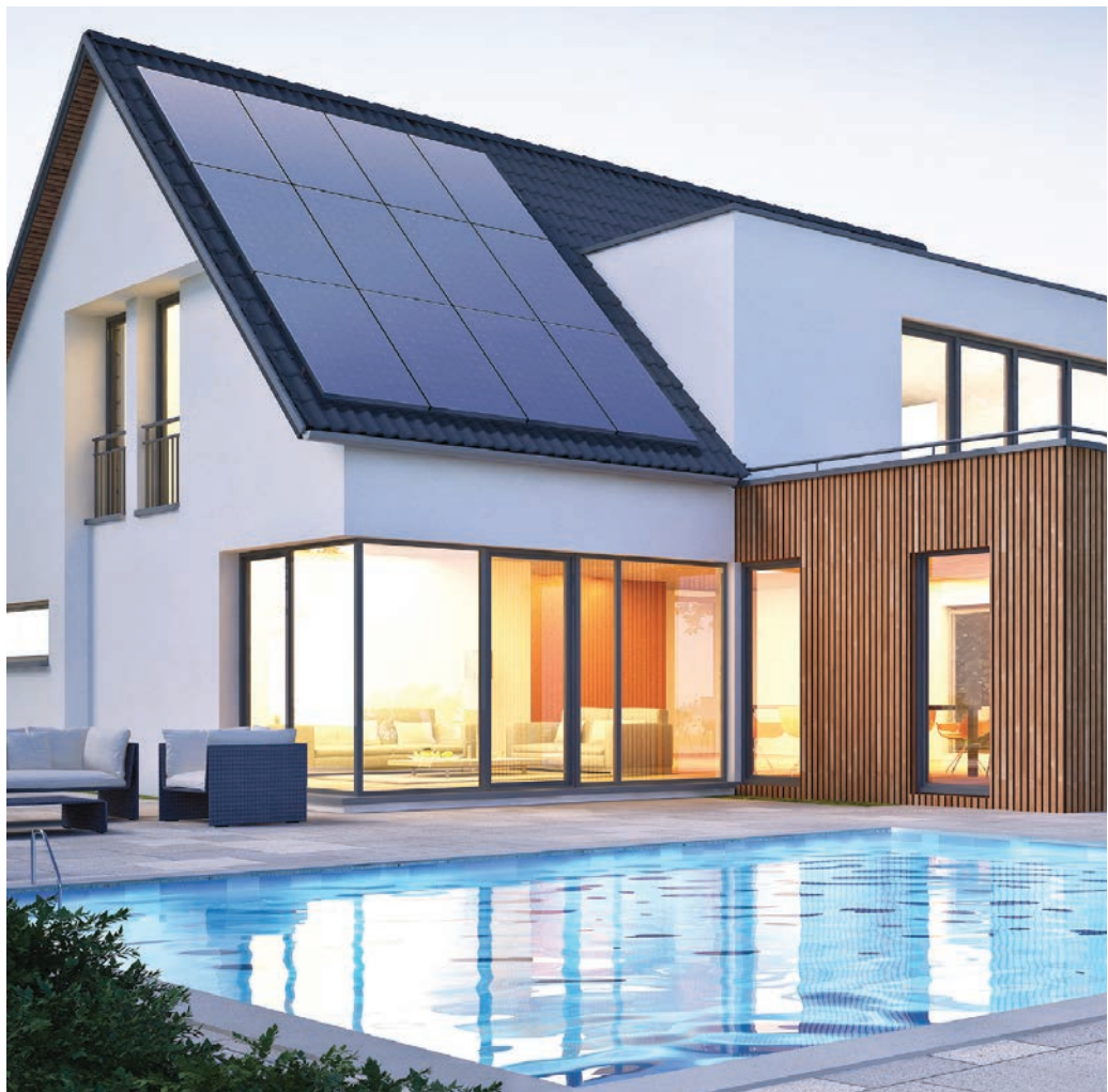
Semper Solaris is a licensed solar and roofing contractor who provides top quality roof replacement and solar installations throughout California.
