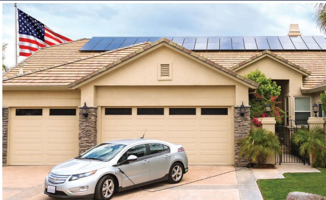
Semper Solaris only uses SunPower panels, designed in America.
