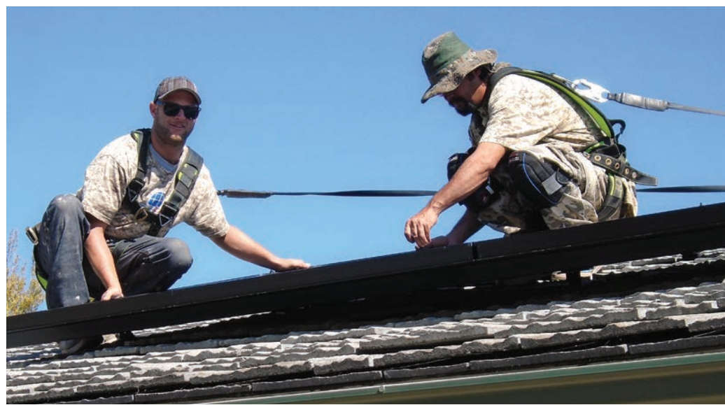
Semper Solaris team installing SunPower panels, which will produce 70% more energy.
